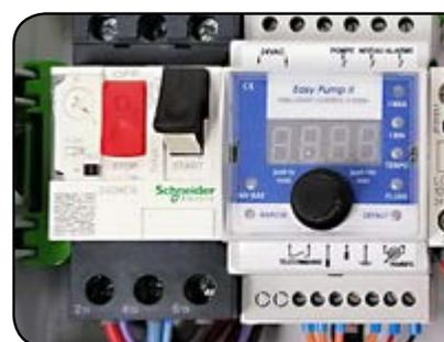
COFFRET D'AUTOMATISME ET DE PROTECTION POUR LA COMMANDE D'UNE POMPE ET D'UN SURPRESSEUR.
